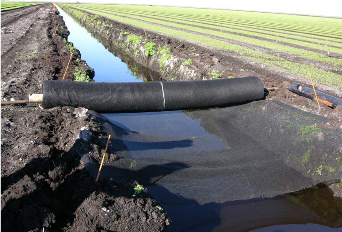
Figure 5. Barrier fence material used in an attempt to cover a lateral canal.
